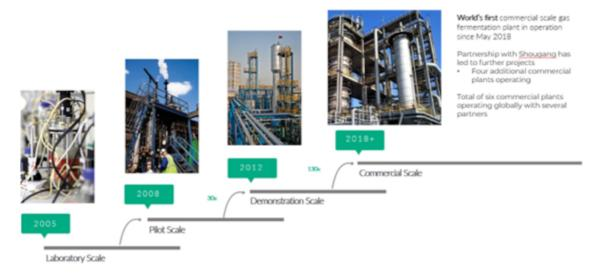
LanzaTech's gas fermentation process has been demonstrated at four sites with 50,000 hours of operation in the field using steel mill waste gases plus another 50,000 hours of operating in the field integrating gasification, gas treatment and gas fermentation. The success of these 100,000 hours of experience at pilot and demonstration scales
