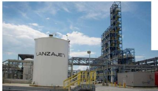
LanzaJet's Freedom Pines renewable fuels refinery will be capable of producing 10 million gallons of sustainable aviation fuel or renewable diesel a year at full capacity.
